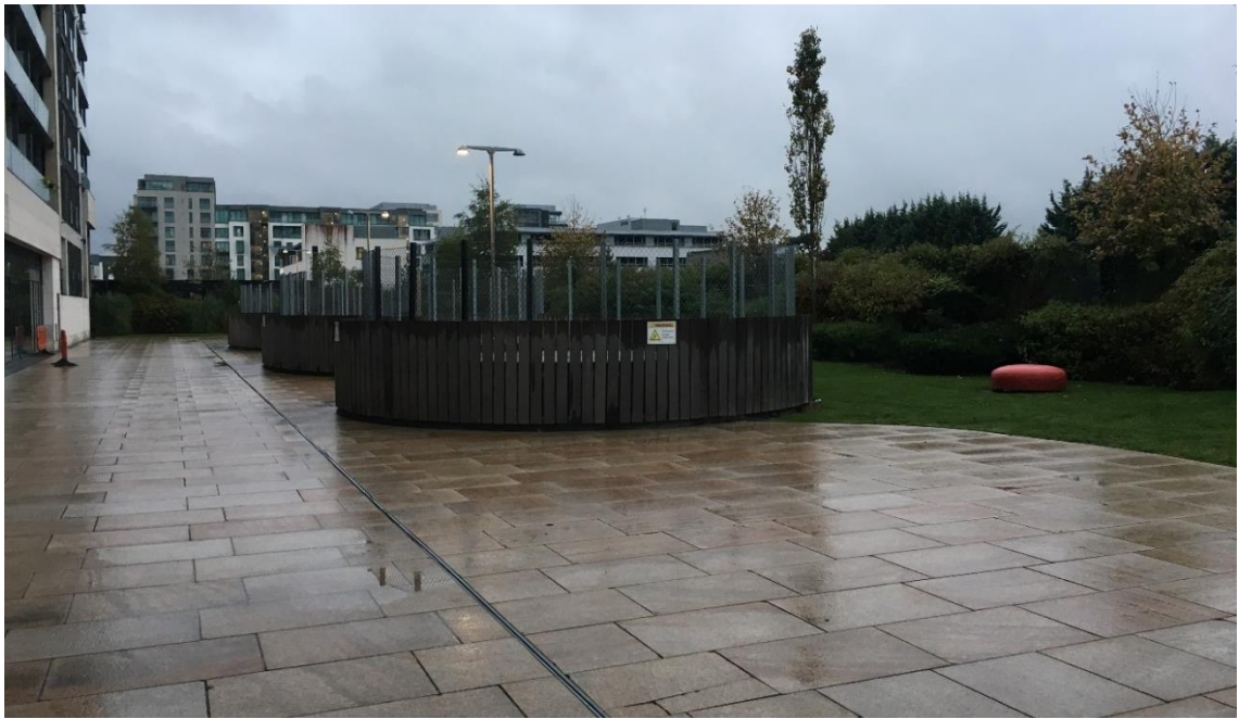
Figure 9.5 – View of existing car park vents to north of site
