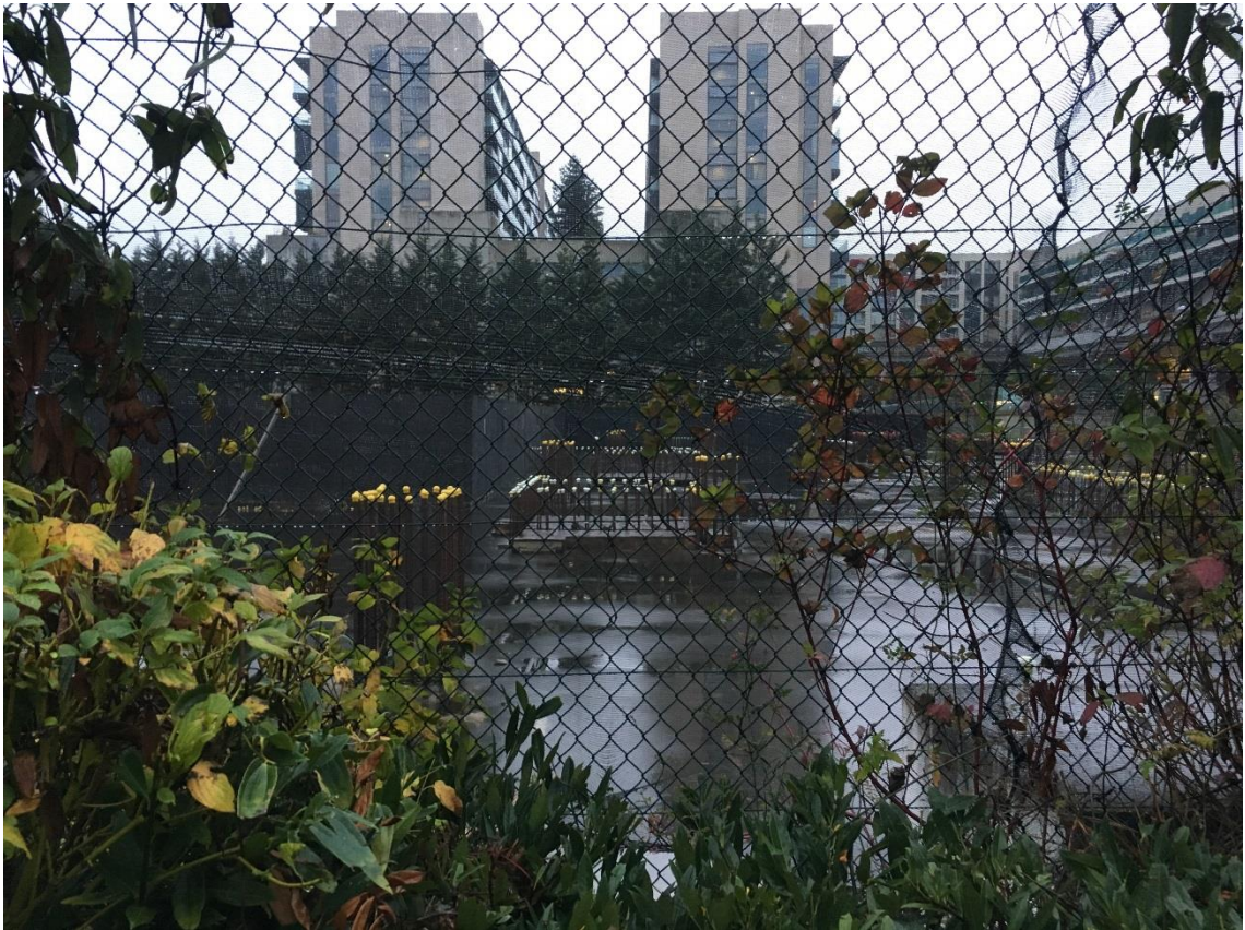
Figure 9.1 – View south into constructed part of site
