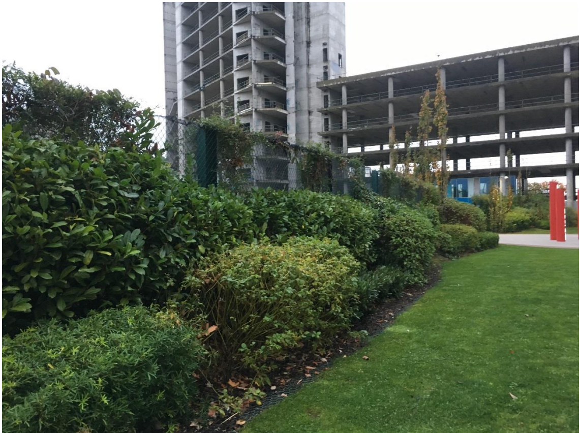
Figure 9.9 – View west towards Sentinel Building (part-complete)
